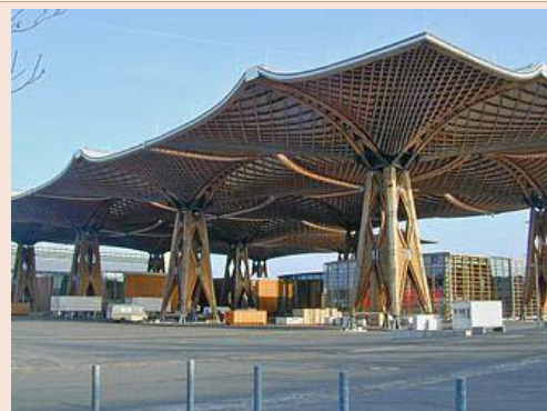
Figure 9: Large self-supporting wooden roof in Hannover, Germany (Bischoff, 2006).
