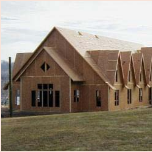
Figure 7: Structured Insulated Panels on the exterior of a residence (Image credits-Murus Structural Insulating Panels).
