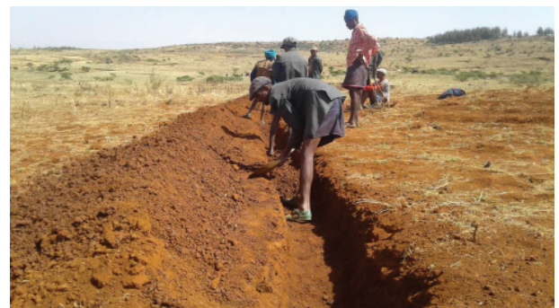
Figure 5: Physical soil and water conservation structure /soil bund/ Sources: - gozamin woreda 2018.
