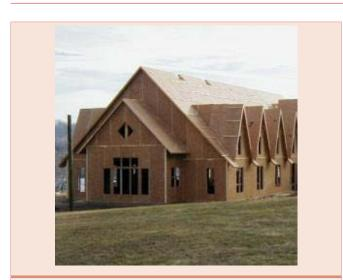
Figure 7: Structured Insulated Panels on the exterior of a residence (Image credits-Murus Structural Insulating Panels).
