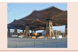
Figure 9: Large self-supporting wooden roof in Hannover, Germany (Bischoff, 2006).
